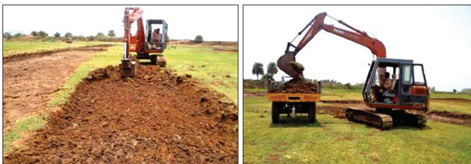
Desilting of tank
