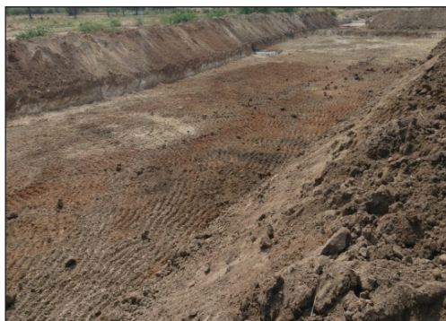
Check dam in Peravali(Anantapur) after desilting
