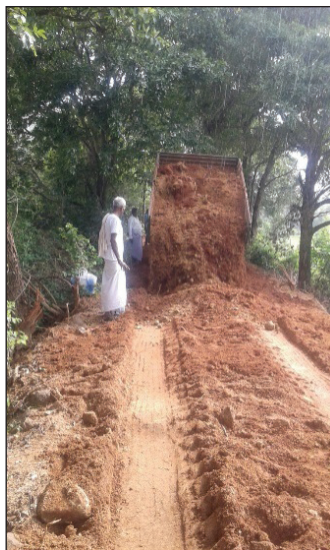
Repair of bund and surplus weir of Chinnakothacheruvu (KVK, Chittoor)
