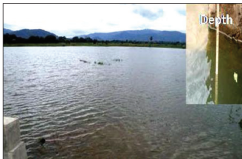
Water level after renovation
