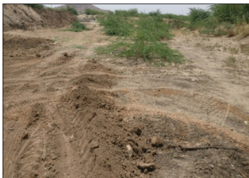
Check dam in Peravali (Anantapur) before desilting
