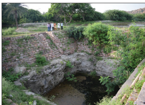
Open well recharged after renovation of the checkdam
