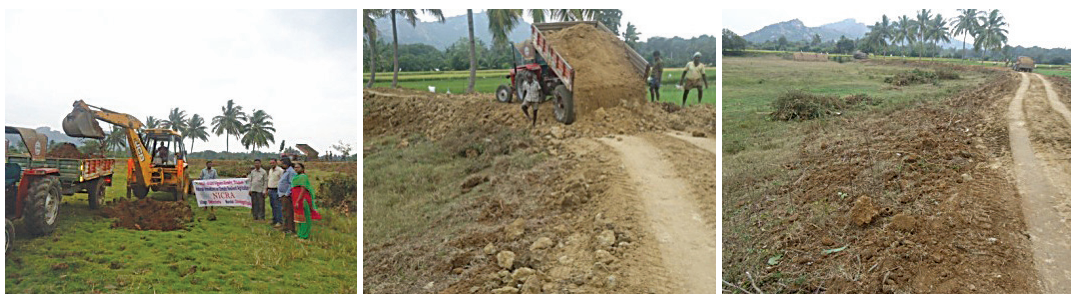
Desilting and strengthening of bund of Errakunta
