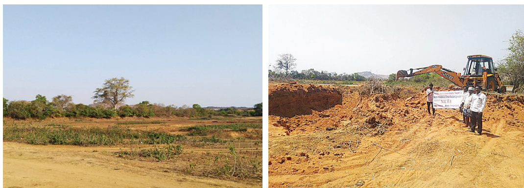
Kamakshammacheruvu before and after renovation
