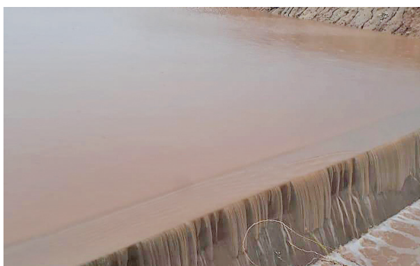
Check dam -1 filled with water after receiving rainfall during September
