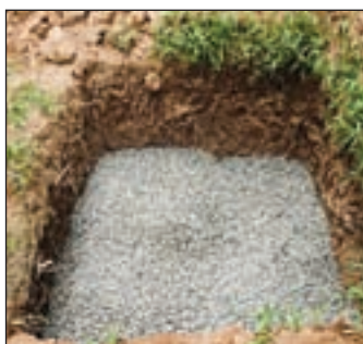
Preparation of bore well recharge pits
