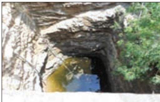
Water level before recharge
