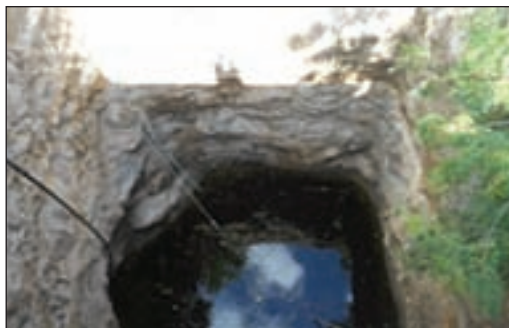
Water level after recharge
