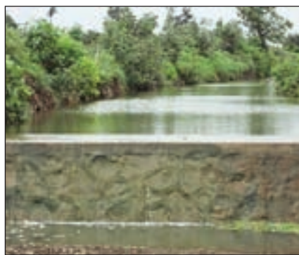
Renovated check dam
