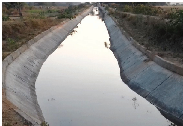
Canal renovation-KVK Gumla mobilised 1.86 crores of money through minor irrigation dept. and MGNREGA
