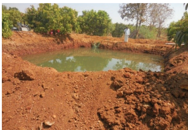
Construction of farm ponds-KVK Davanagere mobilized 25 lakhs from Krishi Bhayga scheme of Karnataka
