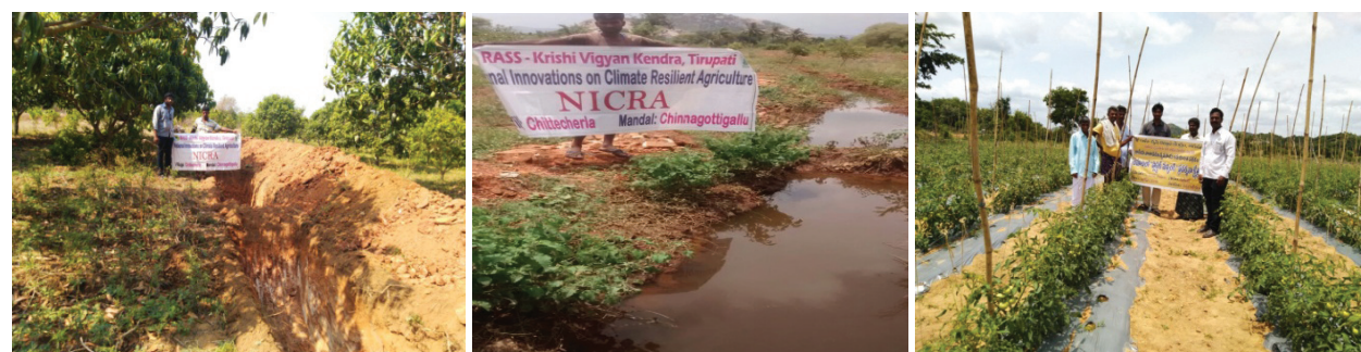
Trench cum bunding and plastic mulching at Chittoor in Andhra Pradesh
